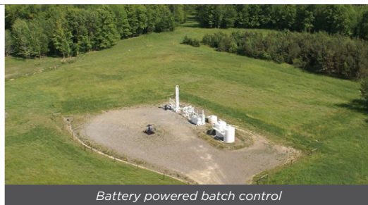
Battery powered batch control
